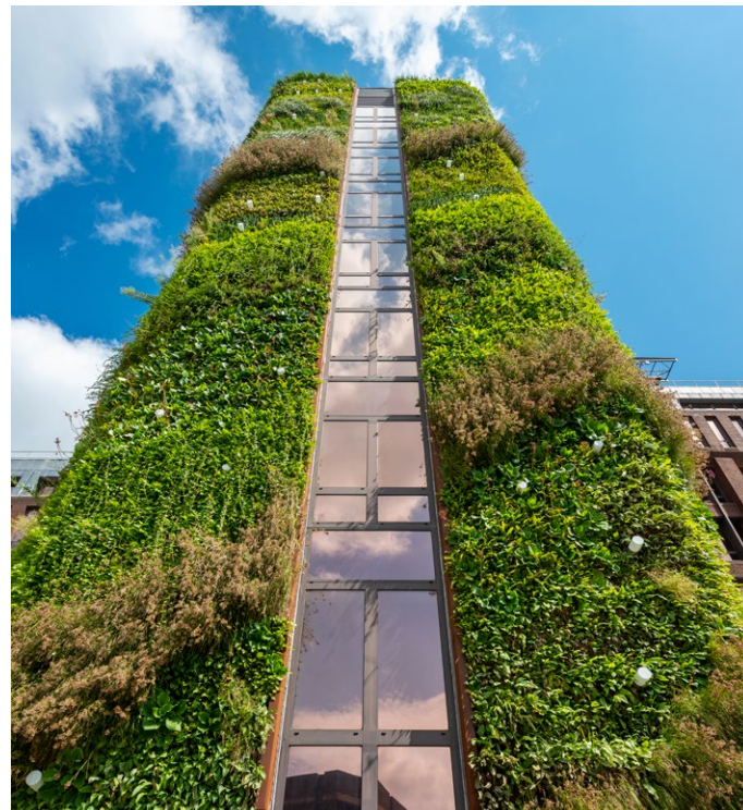
▲ Exterior living 'green' wall
