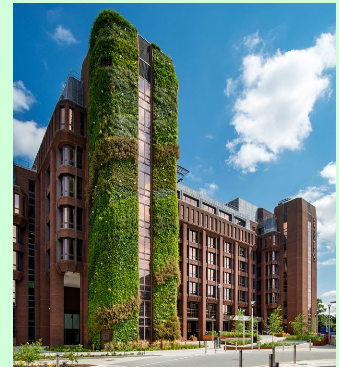
▲ Exterior living 'green' wall
